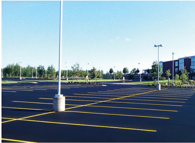
With stores spread out across the nation, it can be difficult for property owners and maintenance managers to create a sealcoating program with the right materials for each site. Pictured here is a freshly sealed parking lot.
